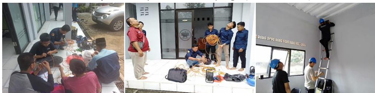
Gambar 1. Proses Instalasi CCTV.
