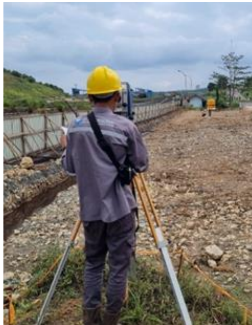
Gambar 6. Penentuan titik bored pile
