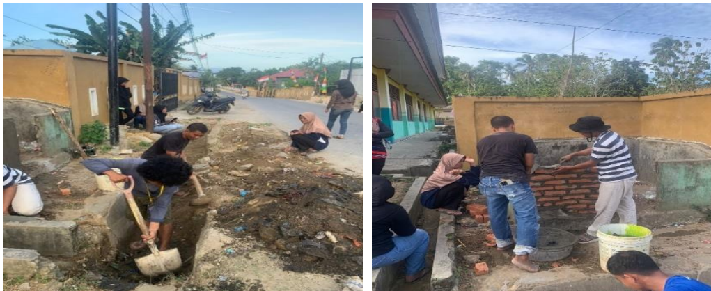
Gambar 5. Proses Pembenahan TPS RT 02
