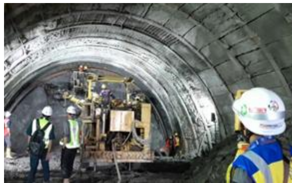
Gambar 5. Setting Steelrib.
