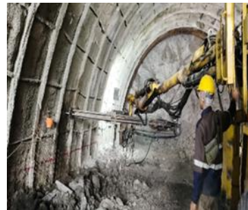
Gambar 11. Drill rockbolt Gambar
