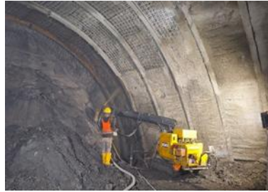
Shotcrete Gambar 10. Shotcrete.
