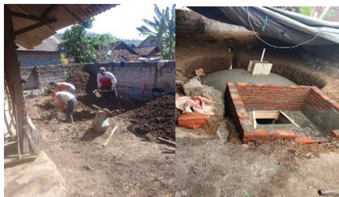
Figure 2. Biogas reactor construction process
